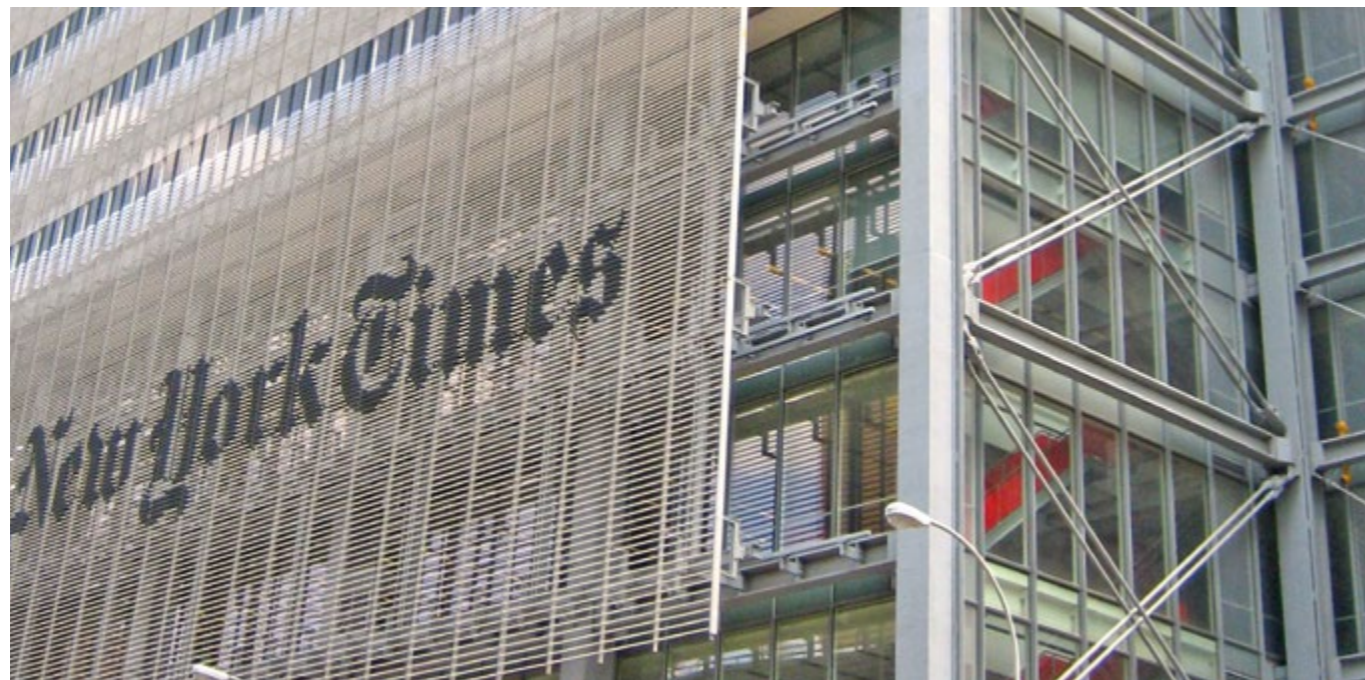
Tandem ASD0540-S bars were used to brace the new 52 floor headquarters for the New York Times newspaper.
