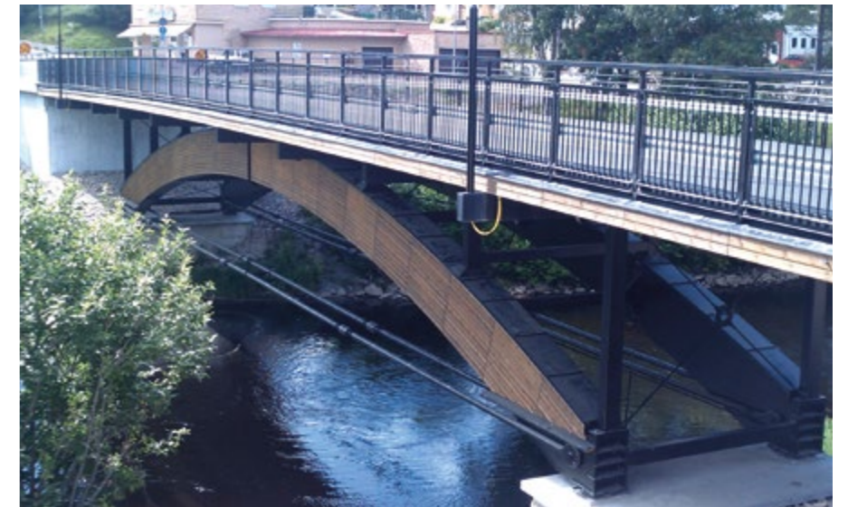
Bowstring trusses, bridges and timber structures
