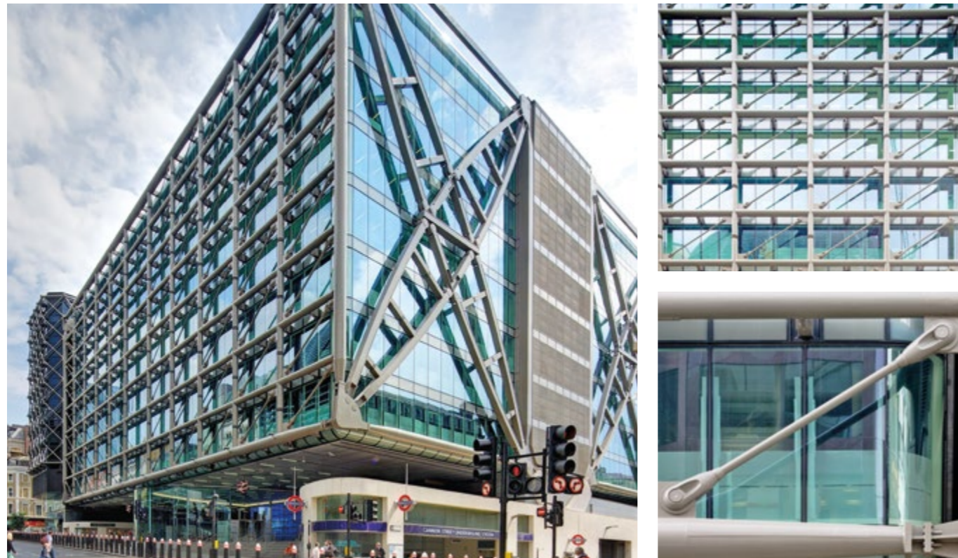
ASD0540-S tie bars M76 to M160 were used as the tension elements in the trusses to form part of this unique and structurally demanding London office building at Cannon Place.
