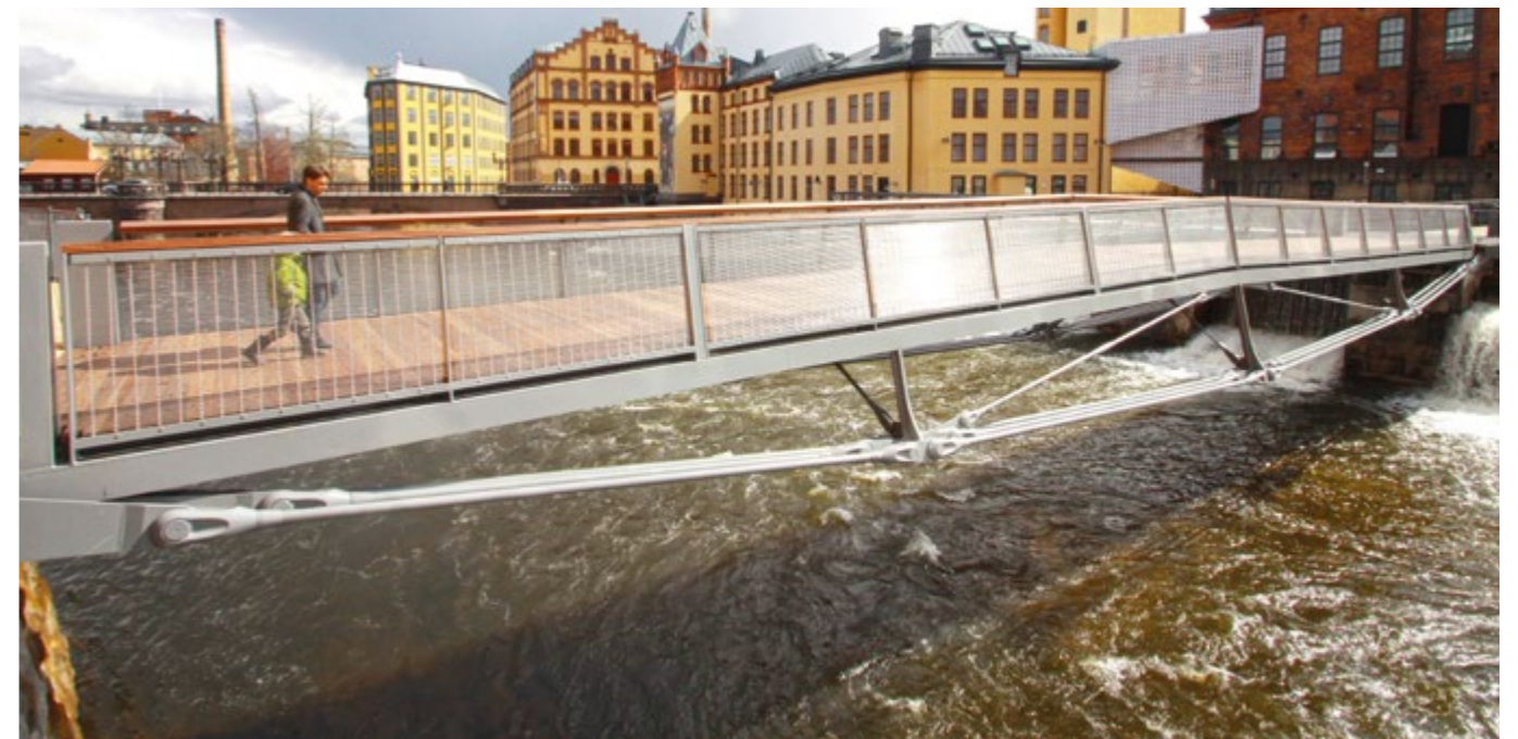
ASD0540-S M56 tie bars were used to form the tension elements for this bowstring truss Kåkenhus footbridge in Norrköping, Sweden.
