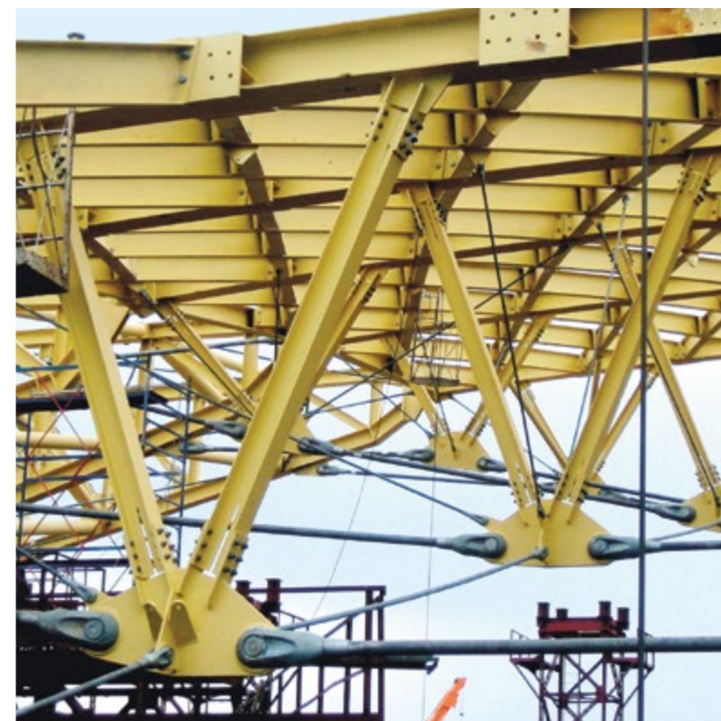
Sheremetyevo airport under construction
