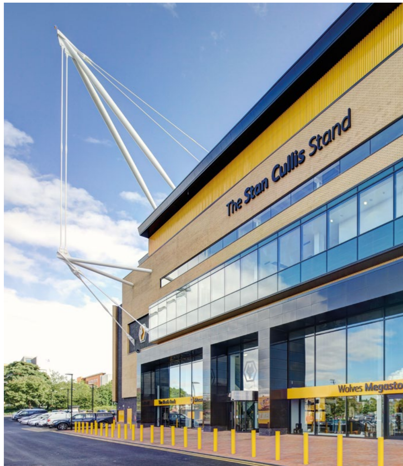
ASD0540-S tie bars were specified for the new stand at Wolverhampton Football Club in the UK as the only system available to support the high loads and be capable of in-situ stressing.
