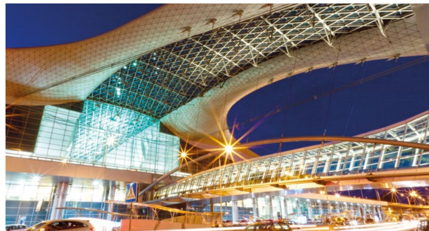
ASD0540-S tie bars are used to support the entrance roof to terminal 3 of Sheremetyevo airport in Moscow.
