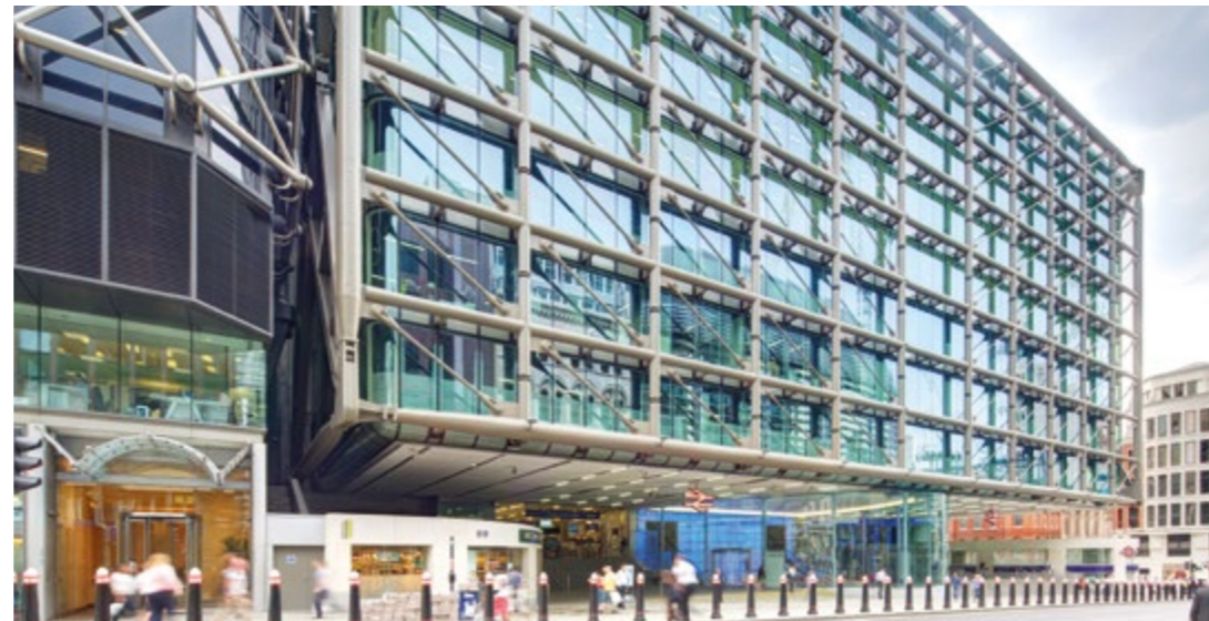
Architectural bracing and facades
