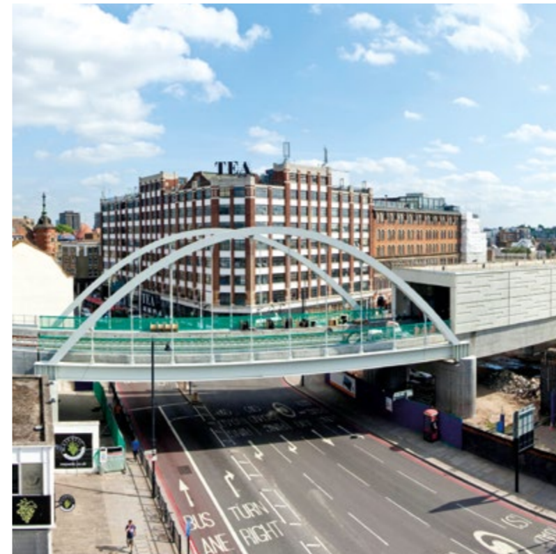
ASD0540-S M90 tie bars are used as hangers on this East London Line railway bridge in Shoreditch. As well as undergoing rigorous QA the system was also fatigue tested to 2m cycles.
